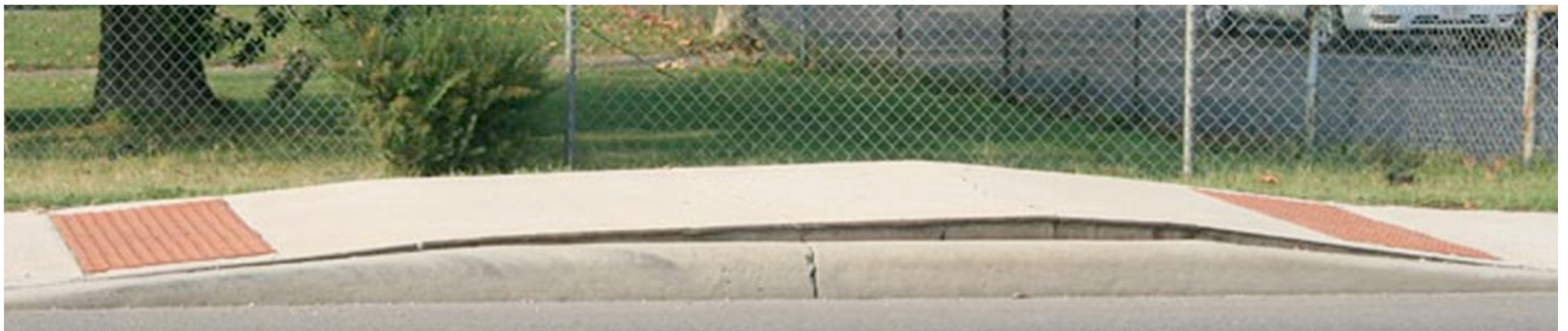
Sidewalk on West Union – T = 33^{\circ}\text{C} ( 91^{\circ}\text{F} ) – expanded about 17mm
