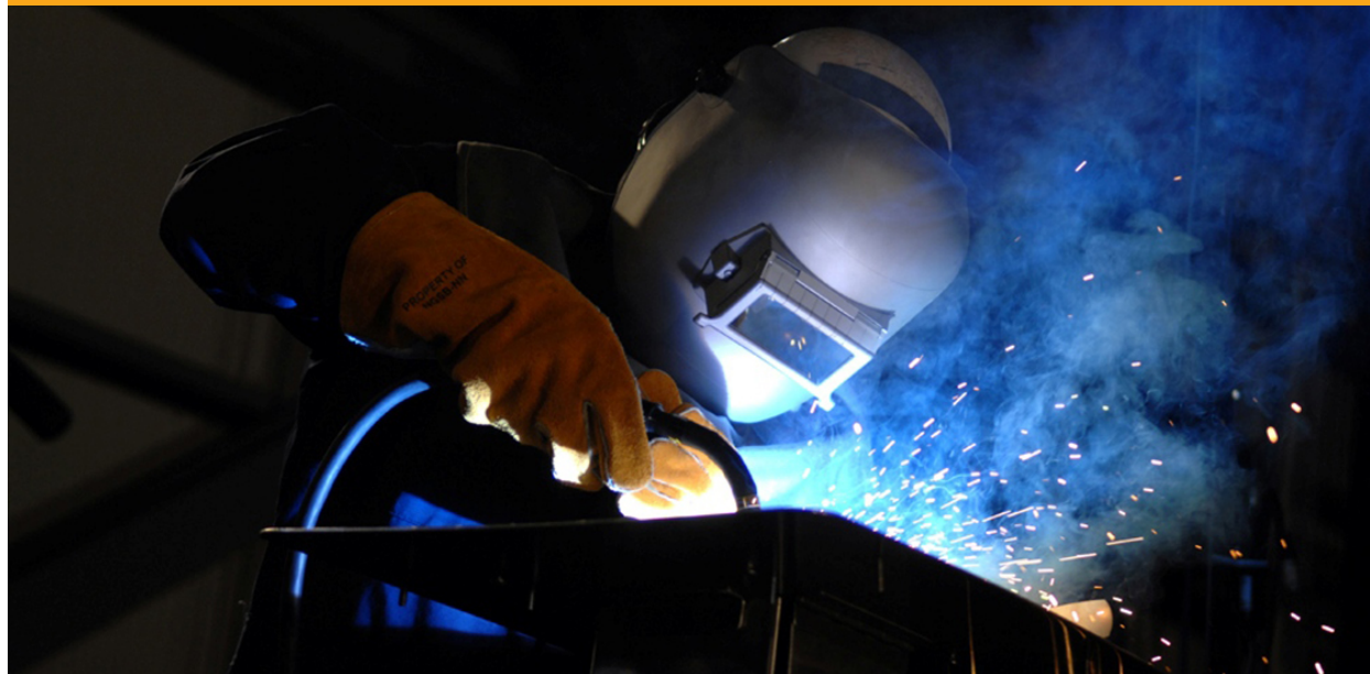
Figure 13.1 The welder's gloves and helmet protect him from the electric arc that transfers enough thermal energy to melt the rod, spray sparks, and burn the retina of an unprotected eye. The thermal energy can be felt on exposed skin a few meters away, and its light can be seen for kilometers. (credit: Kevin S. O'Brien/U.S. Navy)
