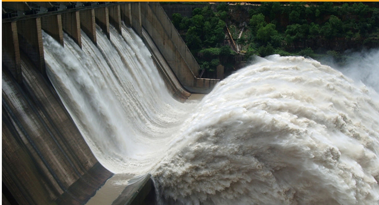
Figure 20.1 Electric energy in massive quantities is transmitted from this hydroelectric facility, the Srisaïlam power station located along the Krishna River in India, by the movement of charge—that is, by electric current. (credit: Chintohere, Wikimedia Commons)
