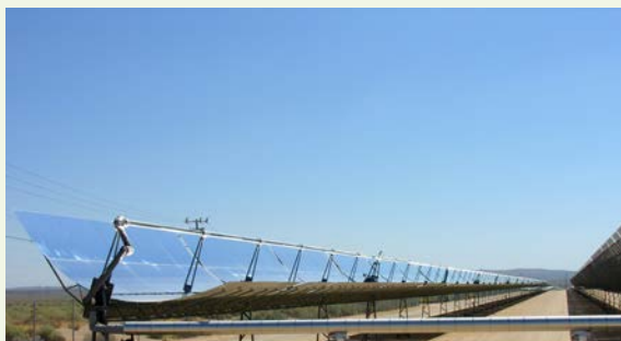
Figure 25.44 Parabolic trough collectors are used to generate electricity in southern California. (credit: kjkolb, Wikimedia Commons)
