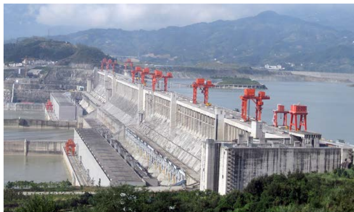
Figure 11.5 Three Gorges Dam in central China. When completed in 2008, this became the world's largest hydroelectric plant, generating power equivalent to that generated by 22 average-sized nuclear power plants. The concrete dam is 181 \text{ m} high and 2.3 \text{ km} across. The reservoir made by this dam is 660 \text{ km} long. Over 1 million people were displaced by the creation of the reservoir. (credit: Le Grand Portage)
